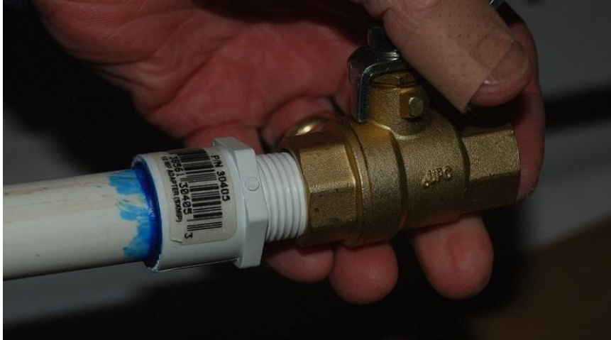
Figure 8. After wrapping the threads of the PVC Male Adaptor (left), screw into the Threaded Ball Valve (right). A wrench may be used to tighten the fitting. Avoid overstressing the glued joints or over-rotating the assembly.
