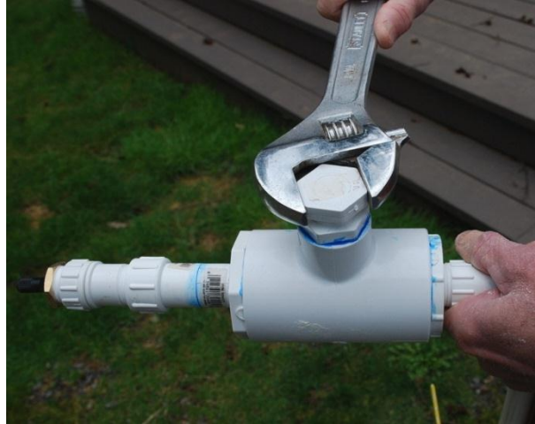
Figure 11. Tighten the Threaded PVC Plug to the T Slip with a crescent or pipe wrench.
